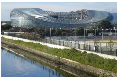
Aviva Stadium Dublin | Ireland
