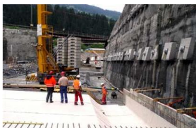
Tunnel Küblis | Switzerland
