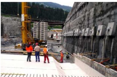
Tunnel Küblis | Switzerland
