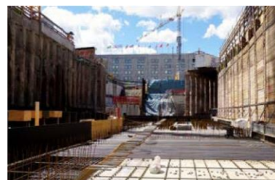
Train Station S21 Stuttgart | Germany
