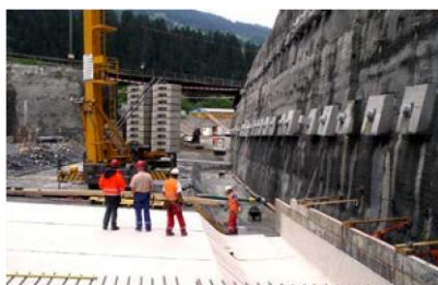
Tunnel Küblis | Switzerland
